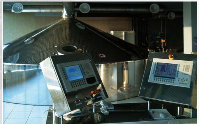
A lauter tub with the boiling house control unit
